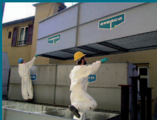
Complete section replacement
