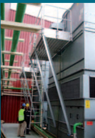
Ladder & Platform Installation
